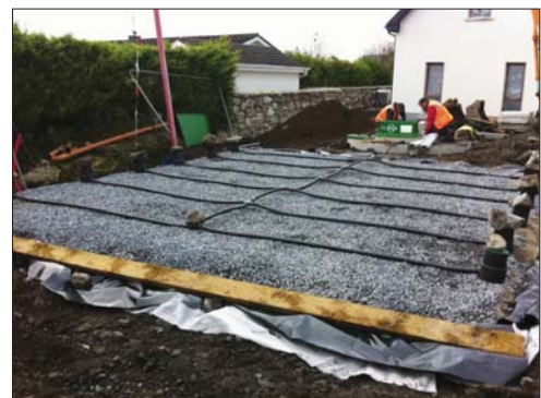
(above) Airtightness plaster behind easi-joints; (above right and below) careful thermal bridging detailing where floor meets external walls; (right) installation of the percolation area for the BioCycle mechanical waste water treatment system; (p47, bottom) triple-glazed argon-filled windows feature heavily on the southern facade to avail of solar gains; (right) ply boxes and stop ends for cellulose insulation, (top) the sheep wool insulated service cavity inside the airtight layer
